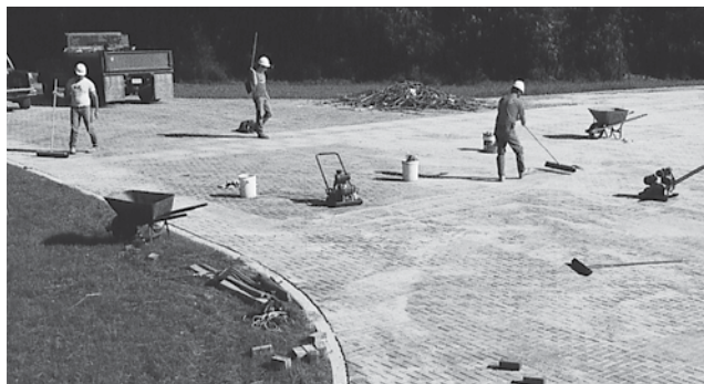
Figure 12. Excess sand swept from the finished surface will make the pavement ready for traffic.
