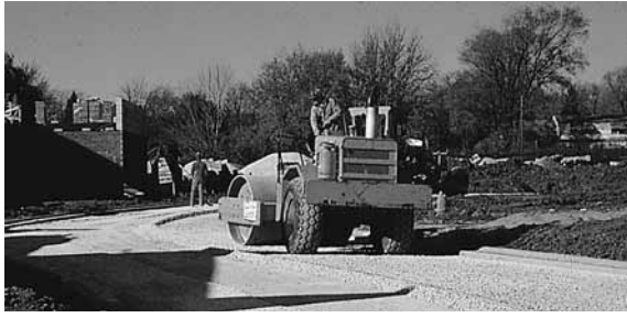
Figure 4. Base compaction with a vibratory roller.
