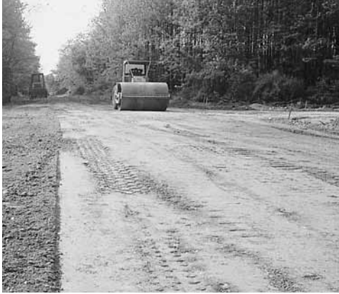
Figure 2. Compacting the soil subgrade.
