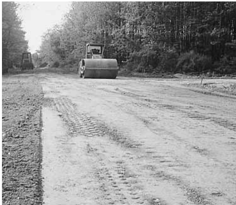
Figure 2. Compacting the soil subgrade.
