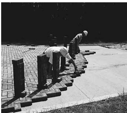
Figure 7. Placing the concrete pavers.
