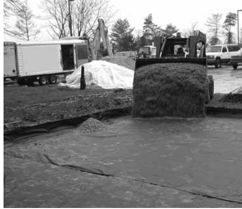
Figure 3. Application of the geotextile under aggregate base.
