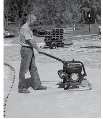
Figure 11. Vibrating sand into the joints.
